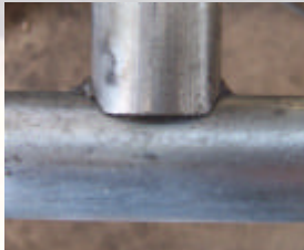
Notched joint prior to welding
